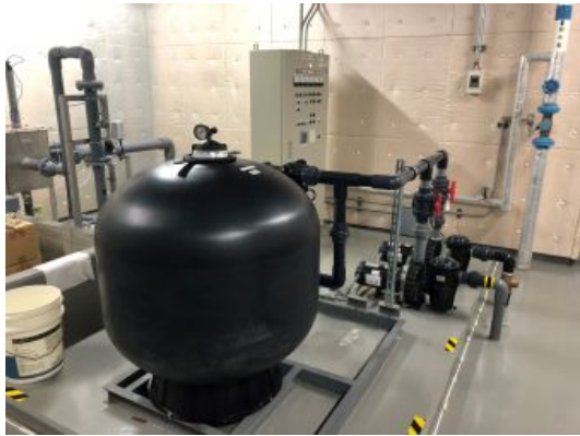
Nifco Head Office Rainwater Filtration System
