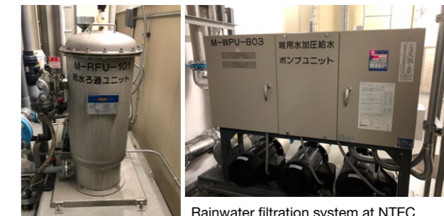
Rainwater filtration system at NTEC
