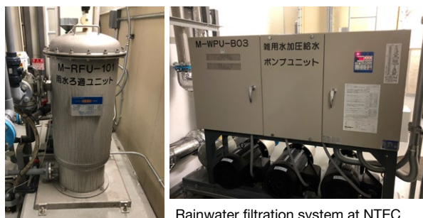
Rainwater filtration system at NTEC
