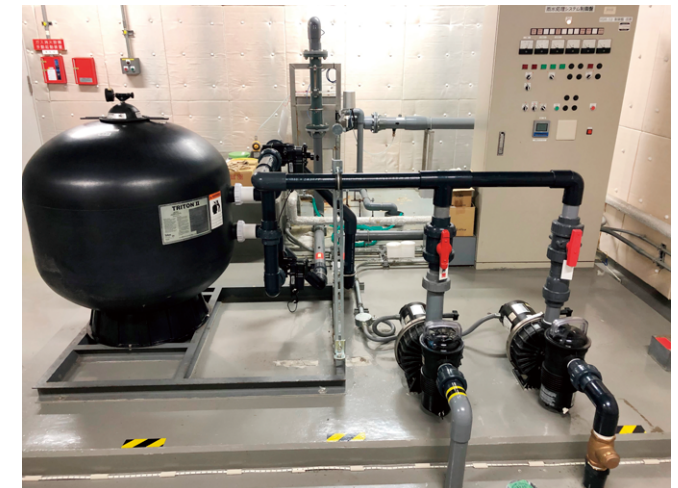
Filtration system (Nifco Head Office)
